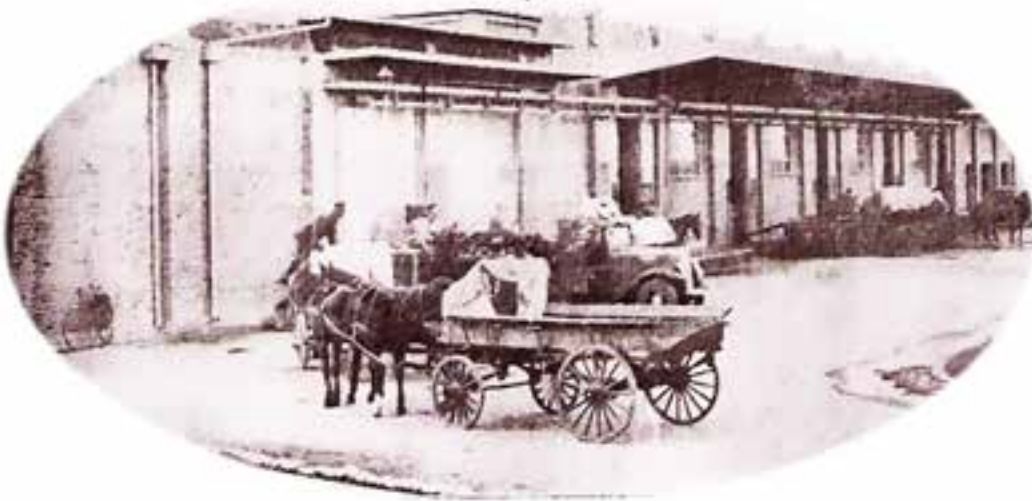
The Abattoir built in 1913. This was to the North of Railway Street and the ruins still remain. (Courtesy Glynis Millett-Clay)
