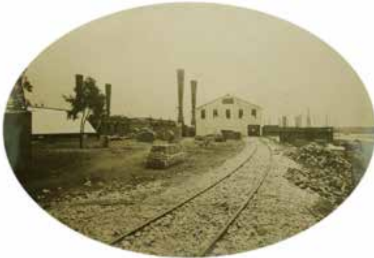
The Benoni Power Station built in 1911 alongside Kleinfontein Dam and abutting Wilstead Street. (Courtesy Peter Wood.)
