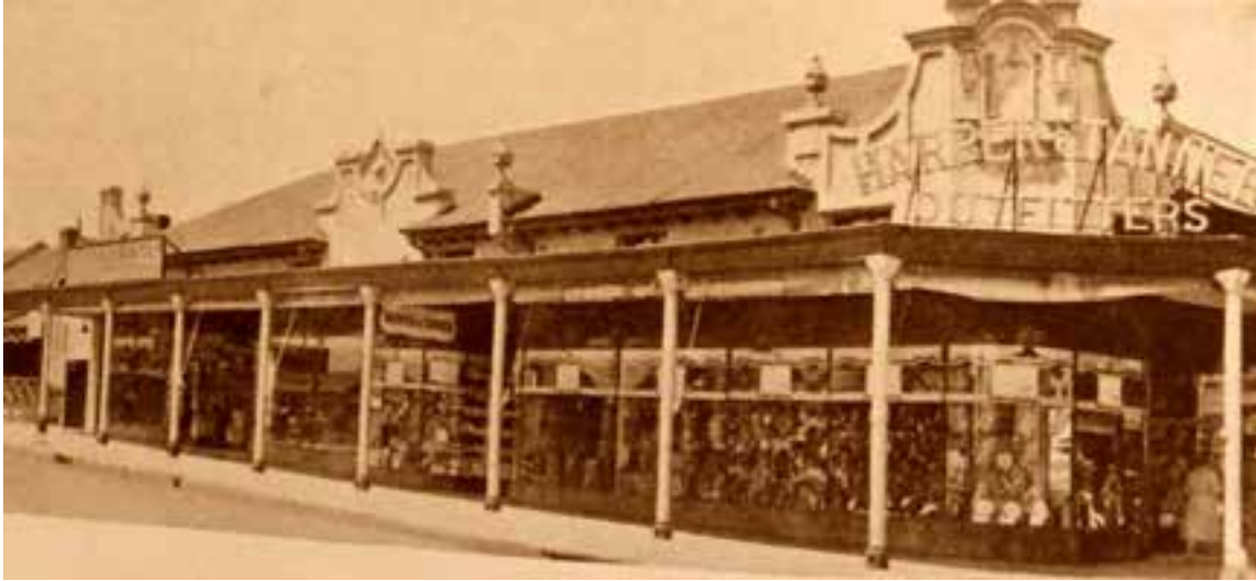
21 Princes Avenue, built in 1912 shown here in the 1930's when it was Harper & Tanner Outfitters. (Courtesy Glynis Millett-Clay)
