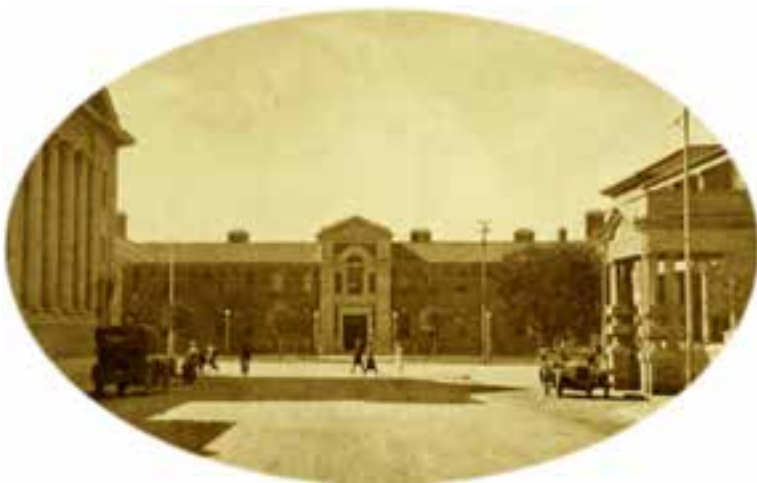
The Municipal Offices in the 1920's taken from Rothsay Street. (Courtesy Glynis Millett-Clay.)
