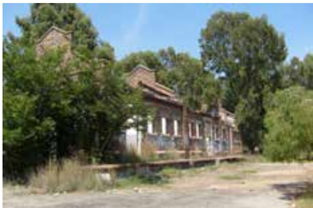
The ruins of the abattoir, north of Railway Avenue.
