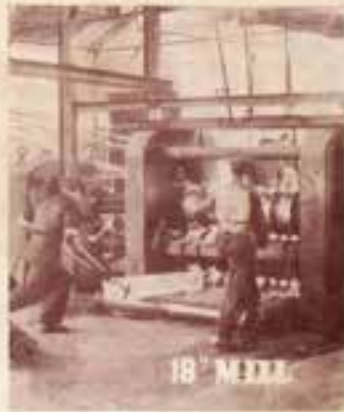
The Rolling Mills at the Dunswart Works
